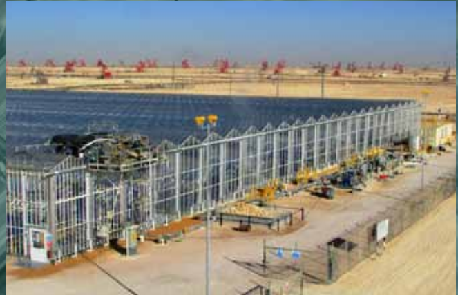
CONSTRUCTION OF EOR STEAM INJECTION PROJECT
