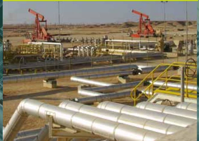
OFF PLOT CONSTRUCTION OF AMAL STEAM SURFACE FACILITIES
