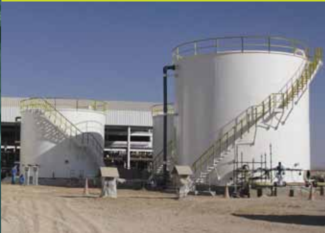
CONSTRUCTION OF TANK FARMS
